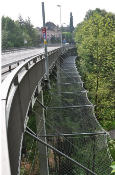
Figure 4 : Filets horizontaux, Rotbachbrücke, Rothenburg
